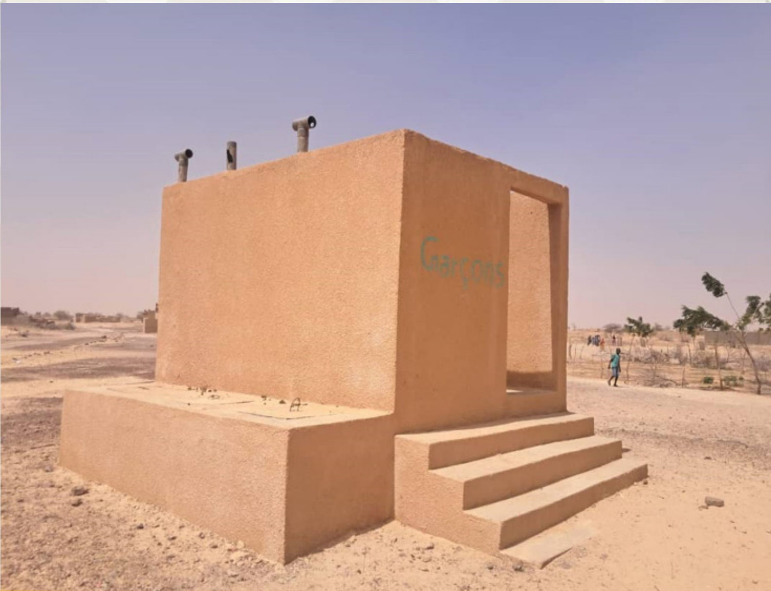
Figure 21: Latrine after rehabilitation
